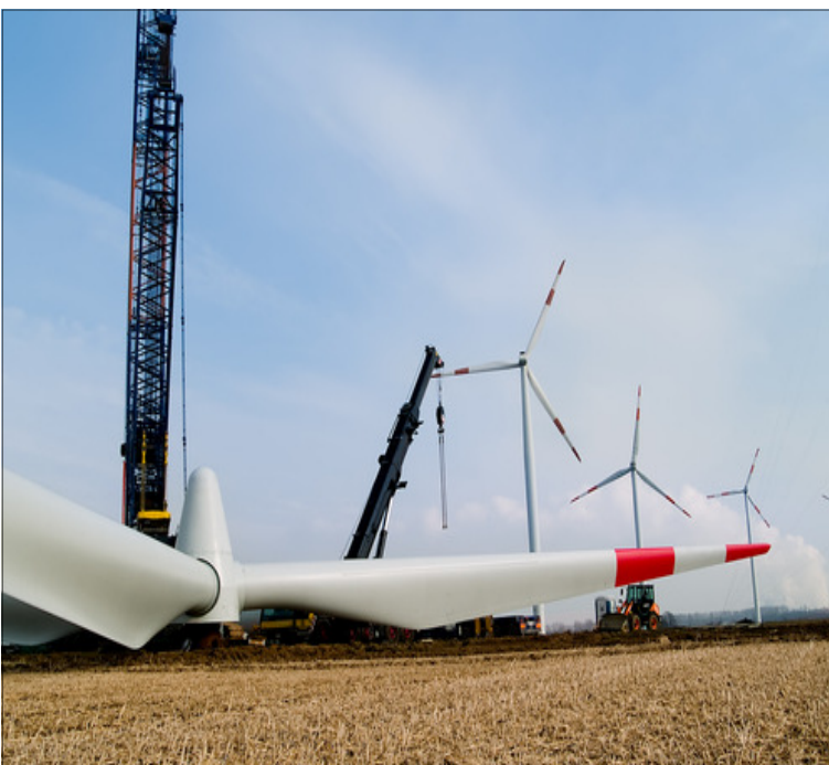
Figure 4. Wind Turbine Rotor and Blades during Assembly
