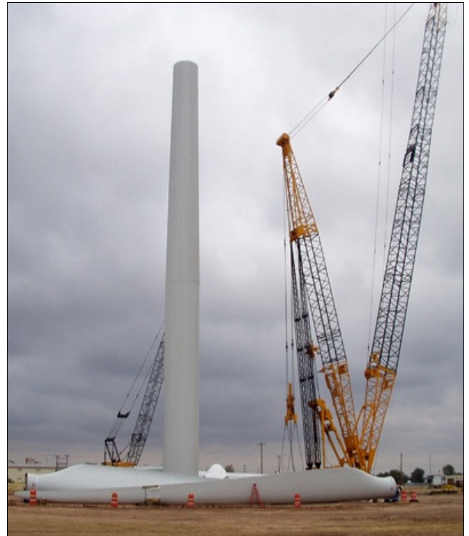
Figure 3. Wind Turbine Construction
